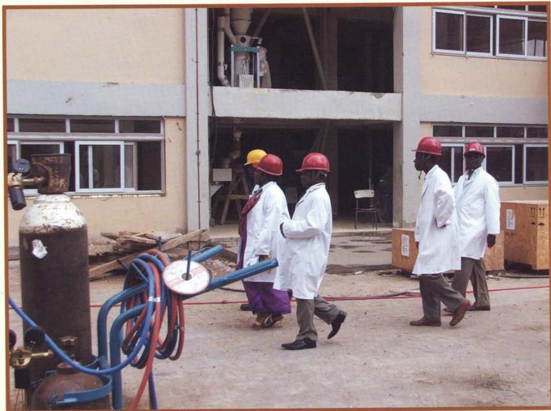
Madam Cecilia Dapaah together with Hon. Stephen Balado Manu, Messrs. David Coleman and Rockson Asare (All Board Members) on visit to the expansion project site.
