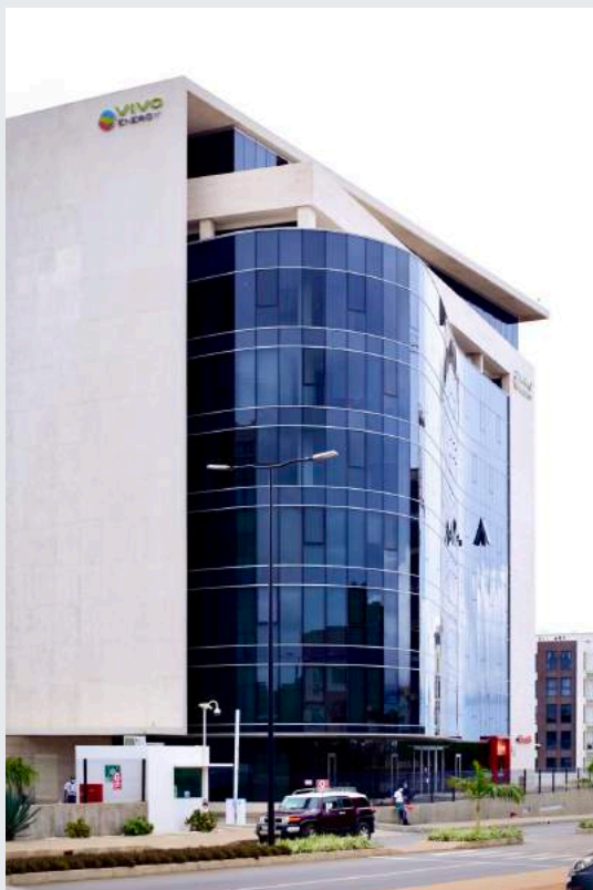
The Vivo Energy Ghana head office located in Cantonments, Accra.
