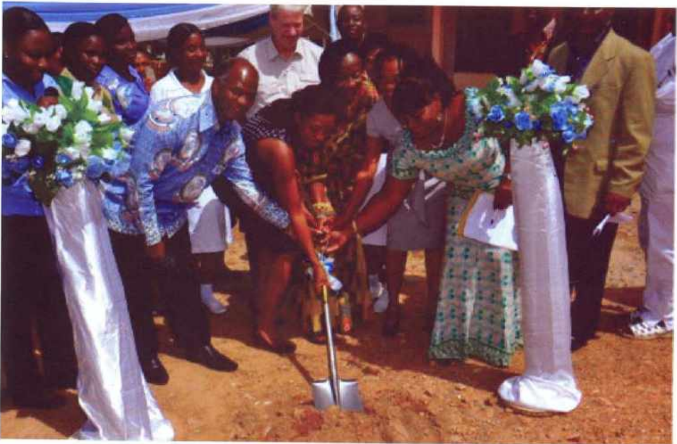
Ms. Sherry Ayittey, Minister of Health breaking grounds for the construction of water delivery system for the Maamobi Hospital. Helping her are Preba Greenstreet, corporate relations director of GGBL and other dignitaries.
