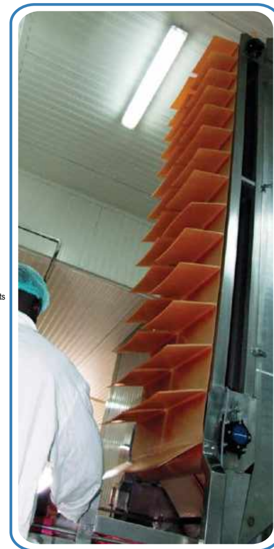
Conveyor belt of spiral freezer.
